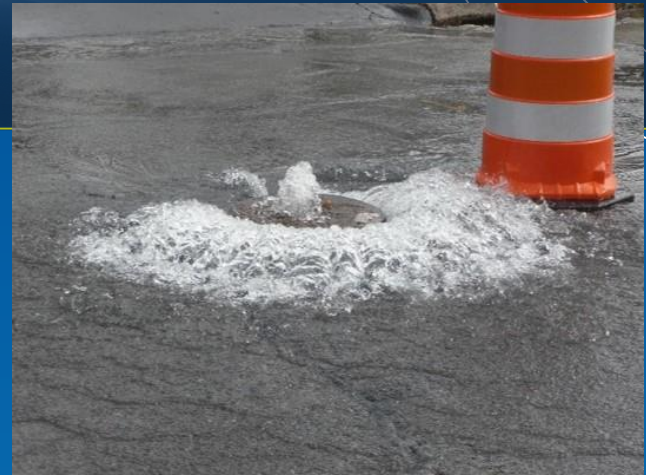
SSO discharged from Manhole
